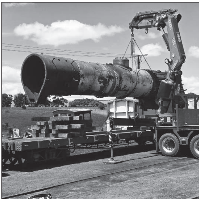
JA1250 boiler and firebox being removed
