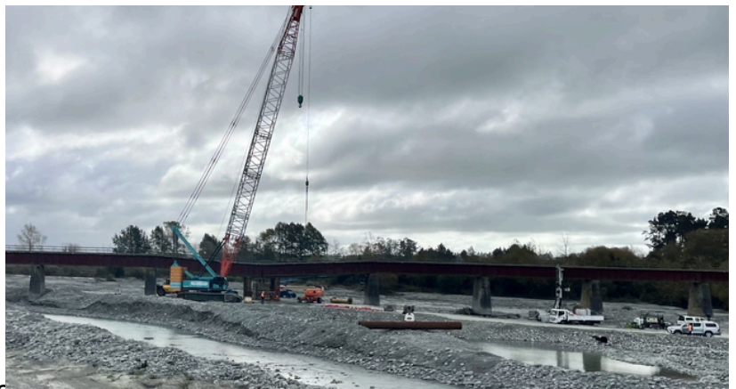
Repair work on the Rangitata rail Bridge in April 2024
