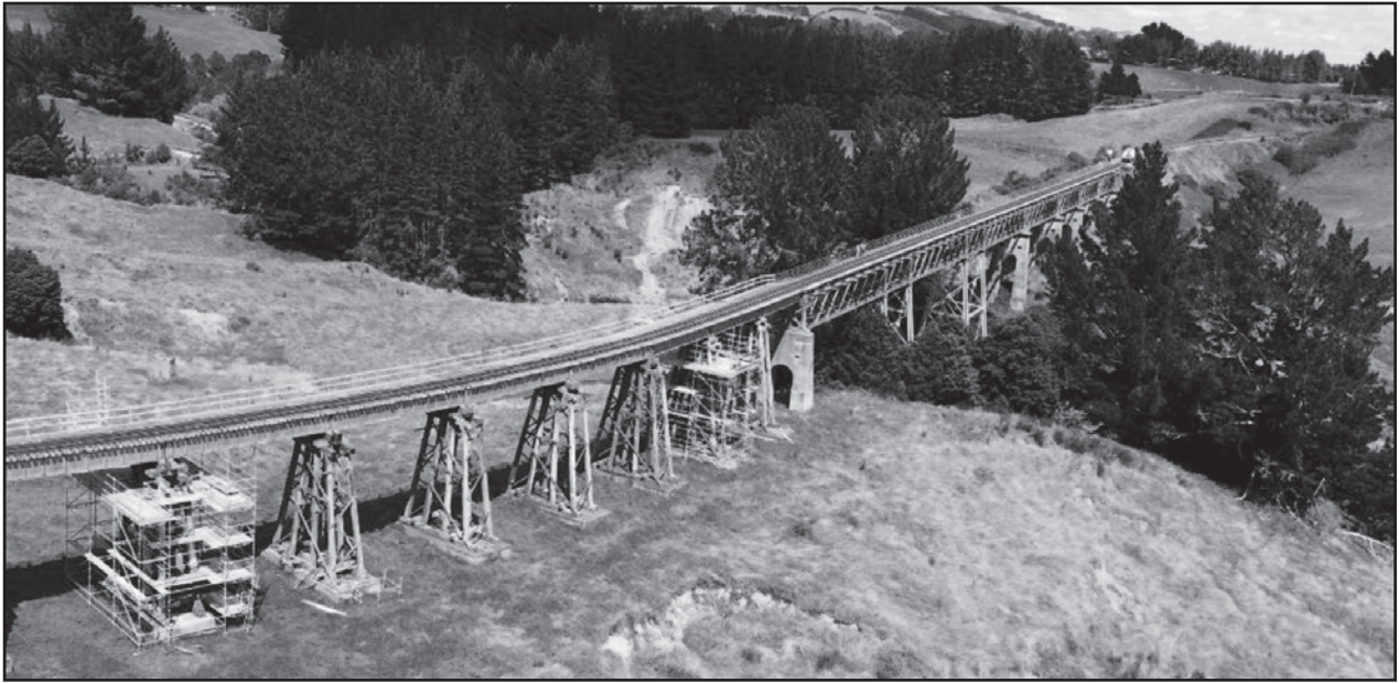
Strengthening work on the Ormondville Viaduct
